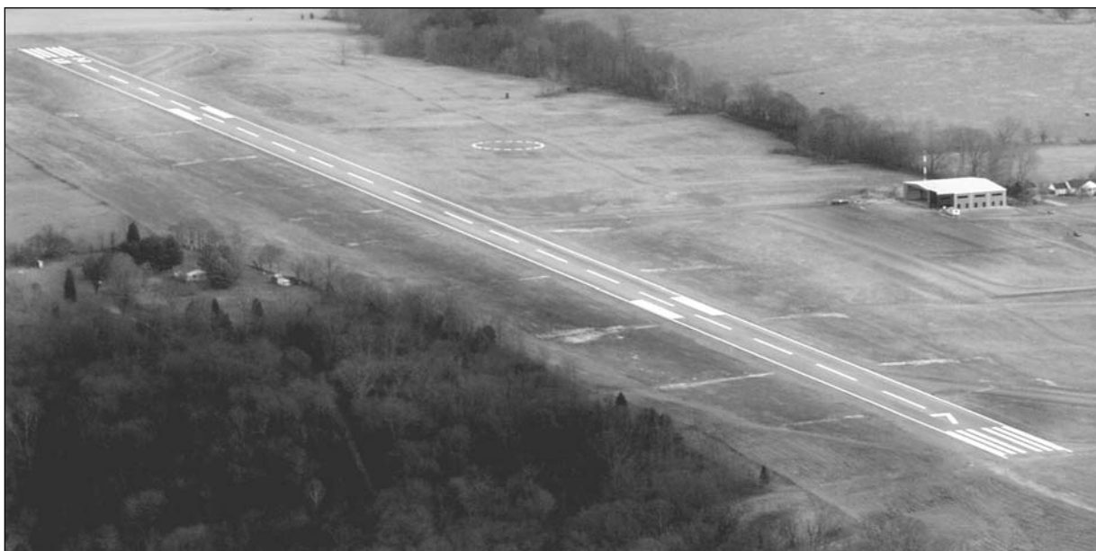
From the air, the Marion Airport's landing strip of just over eight-tenths of a mile, and looks like a race track in front of the hanger and administrative building now under construction.
