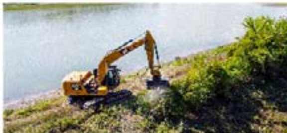
EXCAVATION & FORESTRY WORK
