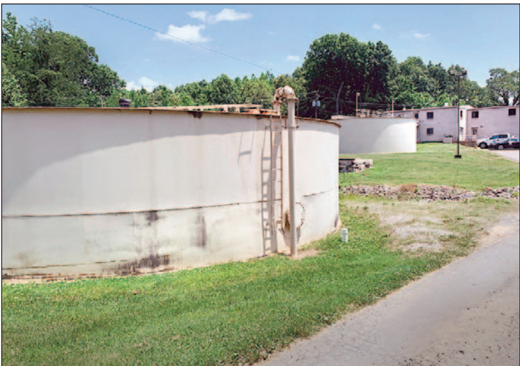
The City of Marion is preparing to rehabilitate and repaint its two clear well water storage tanks at the treatment plant, a project officials say will improve water quality while extending the life of the infrastructure. The $443,000 project will include interior and exterior repairs and painting of the 200,000- and 110,000-gallon tanks, which have not been painted in more than two decades. Water Superintendent Jeff Black said the work will help eliminate accumulated iron and manganese deposits, allowing the tanks to “start fresh.” One tank will remain in service while the other is rehabilitated, with each phase expected to take seven to eight days.
